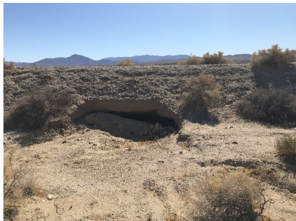
Photograph 9 – Hole at the base of the berm that extends perpendicular through the entirety of the berm (Site 9)
