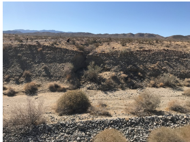
Photograph 4 – Natural gully has eroded earthen berm (Site 4).
