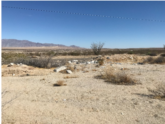
Photograph 7 – Riprap has been filled with sediment (Site 7).
