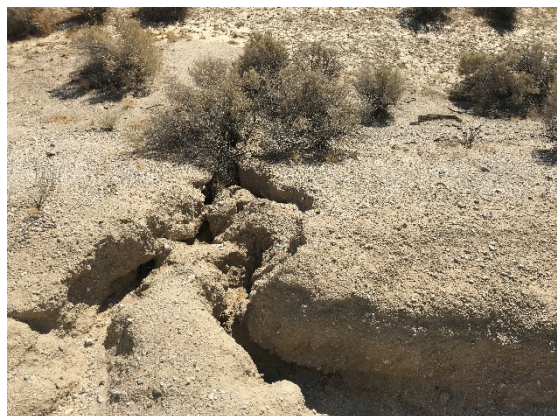
Photograph 15 – Gully erosion in earthen berm (Site 17).
