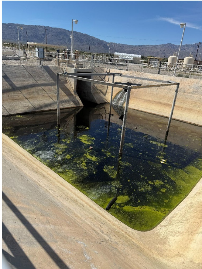
Figure 19. The effluent equalization basin with the remnant metal frame shown.
