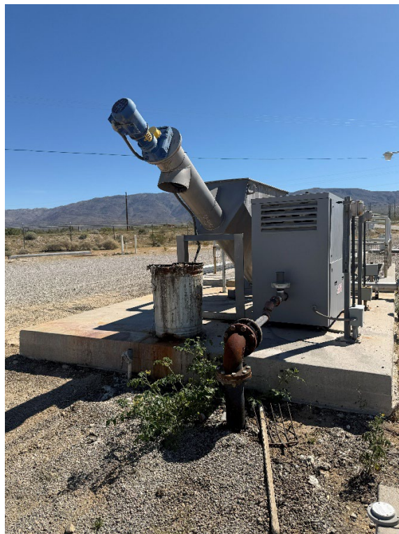
Figure 10. Grit chamber unit with the trash can/grit bin used to collect screenings.
