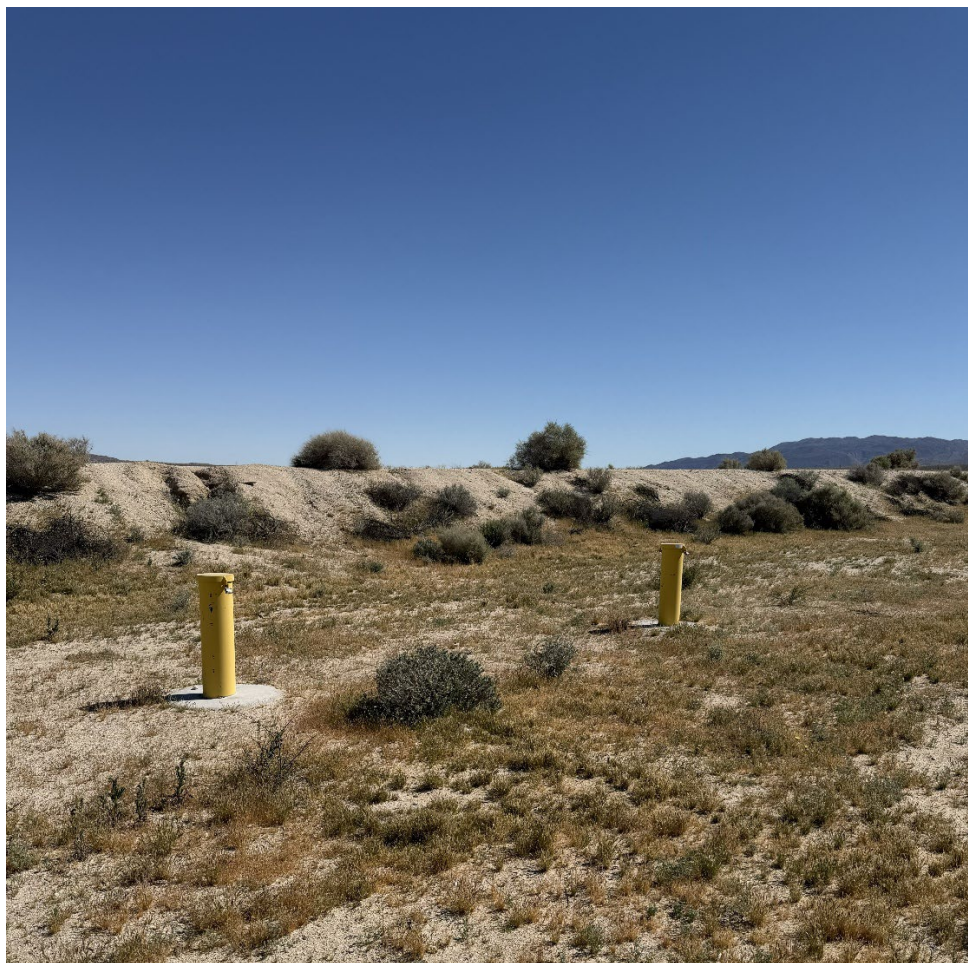
Figure 24. Two of the groundwater monitoring wells inspected. The wells are properly locked.
