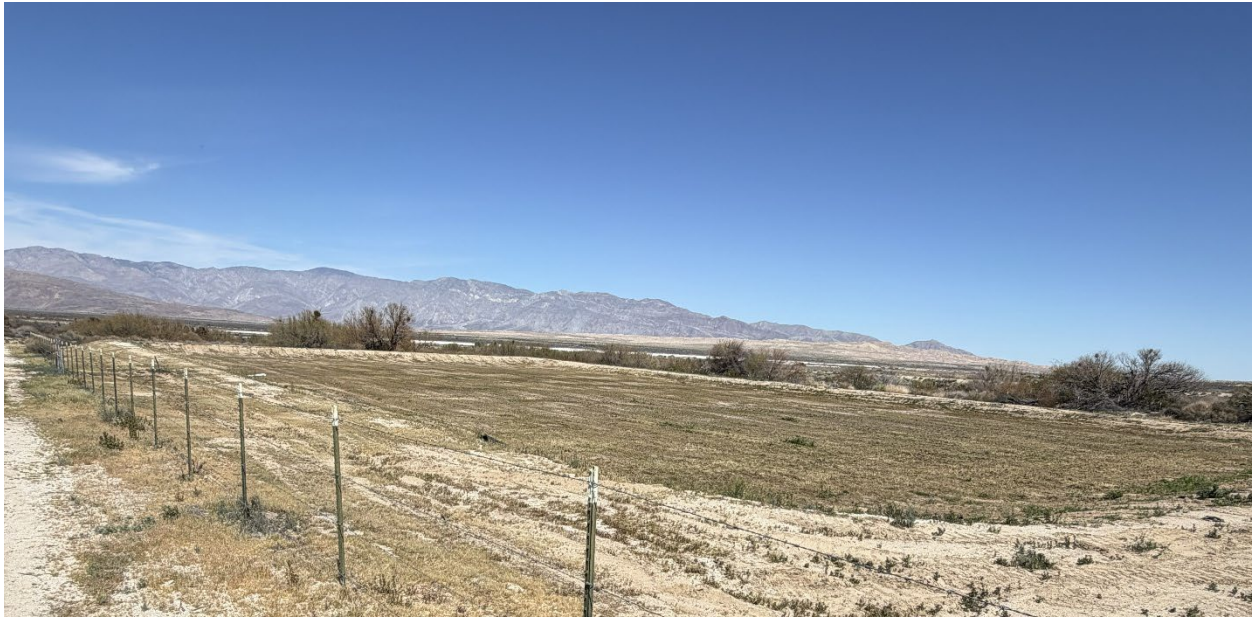
Figure 23. The second evaporation/percolation pond not in use at the time of inspection.
