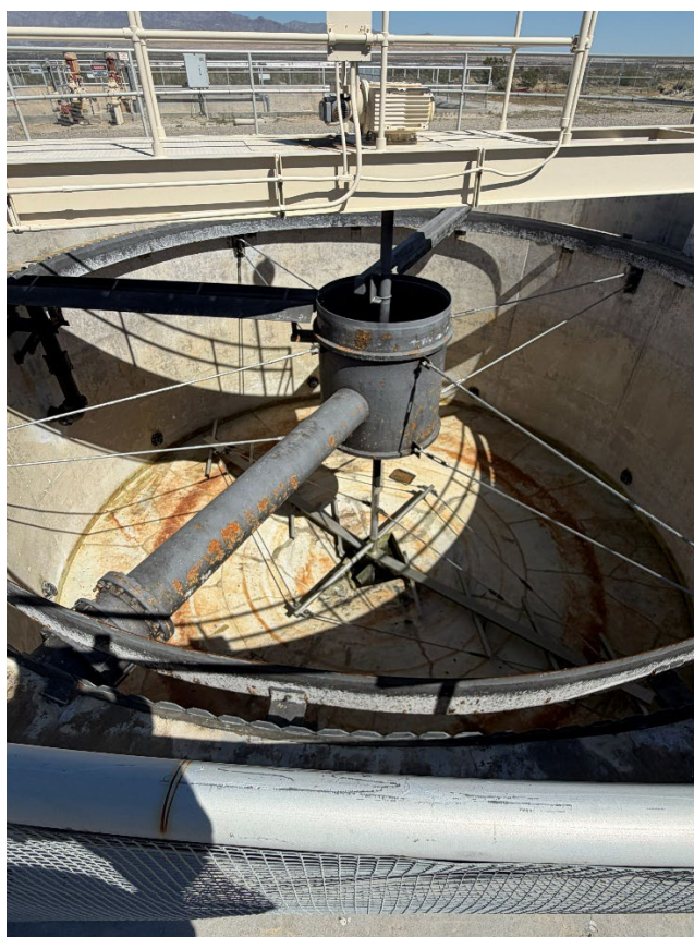
Figure 18. Clarifier 2 not in use at the time of inspection.
