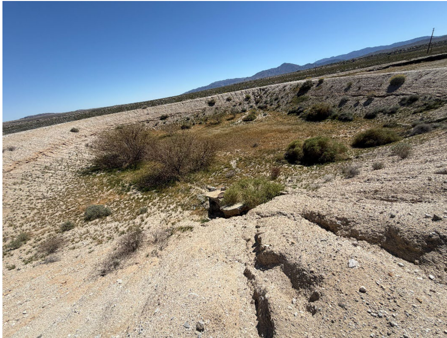
Figure 21. Emergency standby basin located east of the equalization basin.
