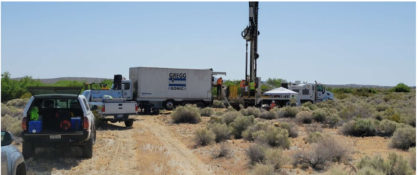
Drill site setup
