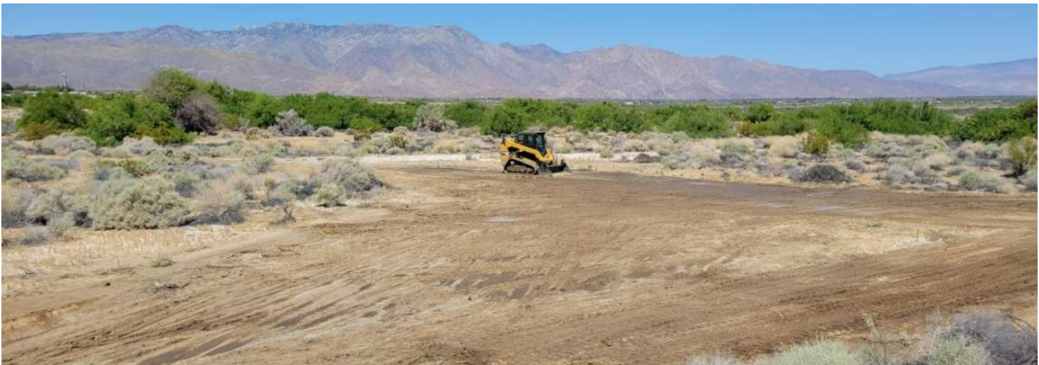
Pre-Construction preparations for WWTP Monitoring Wells site
