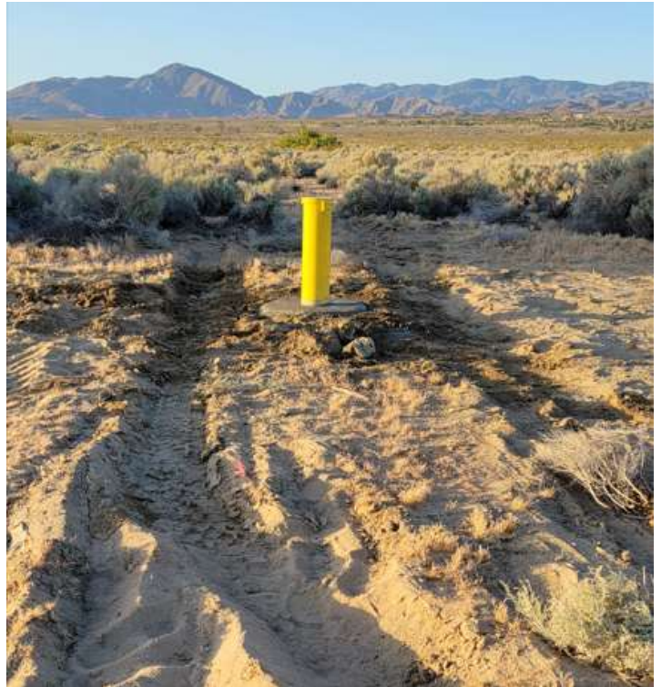
Completed WWTF-2 monitoring well
