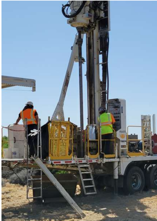
Gregg's Drilling crew monitoring equipment
