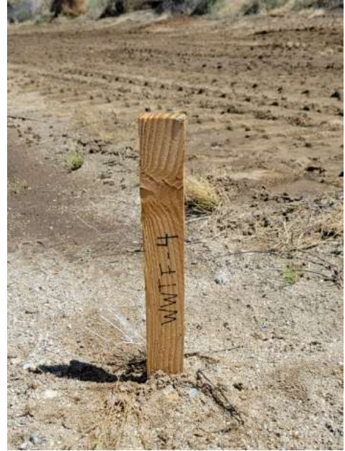
Survey marker indicates drilling location for well WWTF-4
