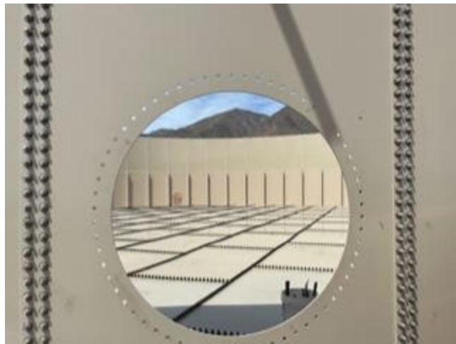
Figure 2 – Construction Progress as of May 2, 2023
