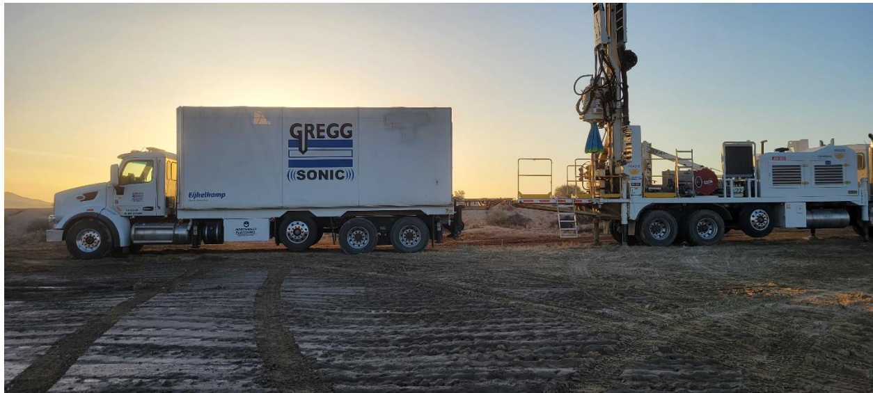
Gregg Drilling preparing to begin work on April 27, 2023
